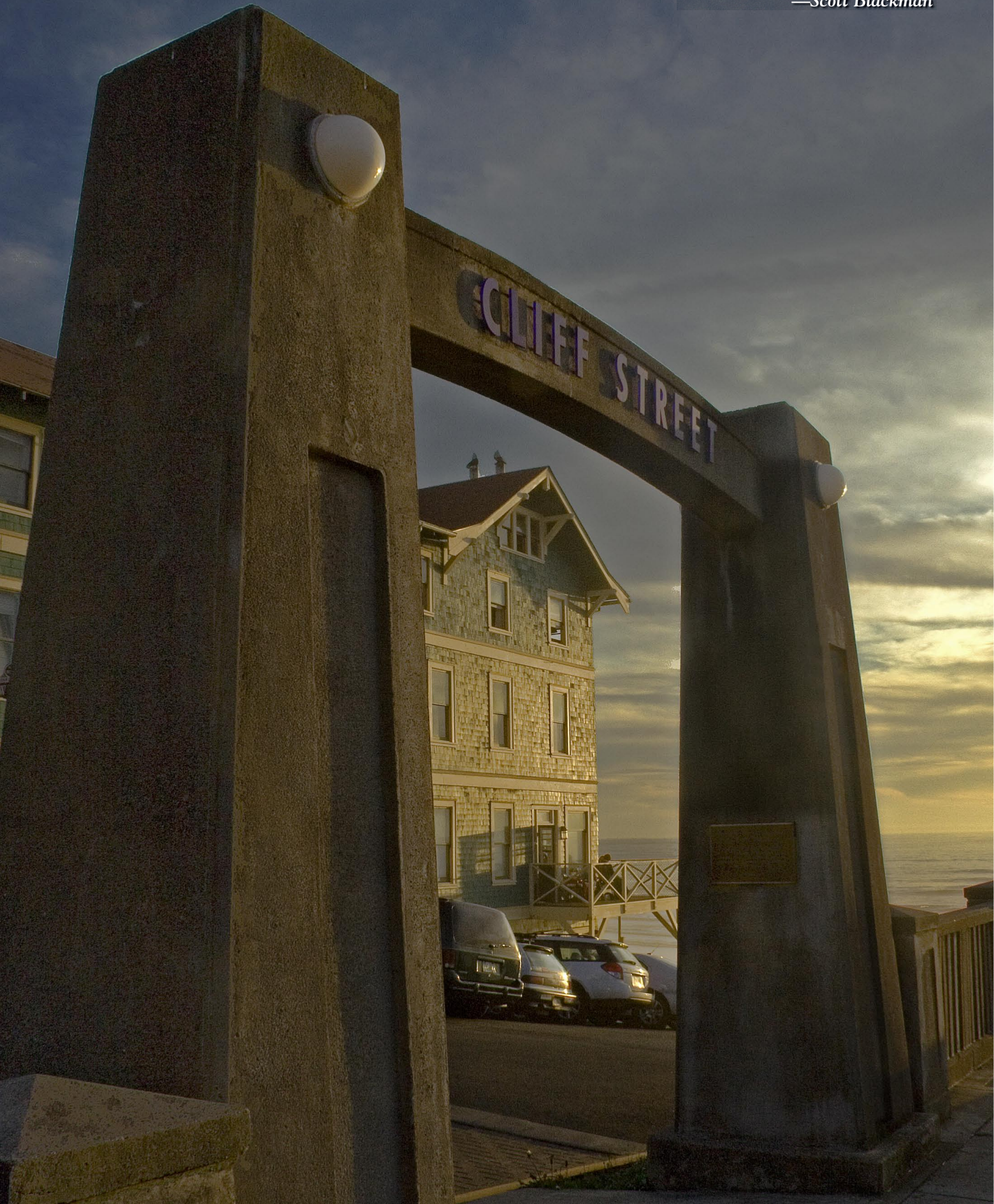
Concrete arch and Sylvia Beach Hotel at Nye Beach, Newport. —Scott Blackman
